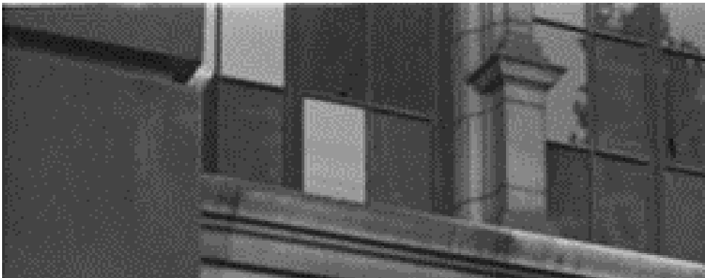
Figure 13, Closeup of Fig. 12. White panes on the left hand side are most likely panes of wartime 'R' glass, coarser and more opaque than traditional glass panes.
