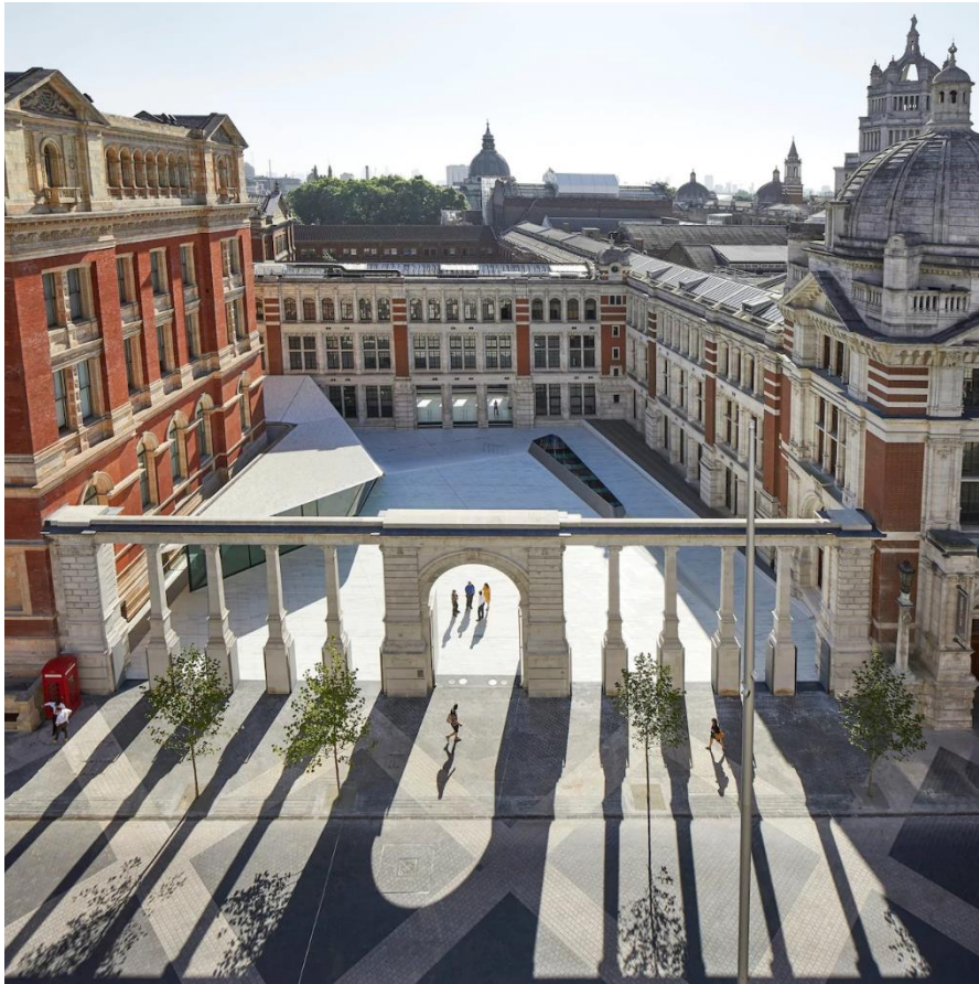
Figure 21, Aerial photo of completed AL_A Sackler Courtyard with gates open. The café sits to the left within the porcelain tiled courtyard. Three incisions made into the museum's Western range are visible towards the back of the image.
