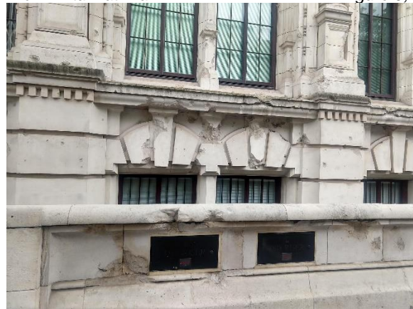
Figure 10, Photo of V&A bomb damage on Exhibition Road, significantly less serious and dramatic in comparison with the previous two depictions of blitztime London in Figures 8 and 9.
