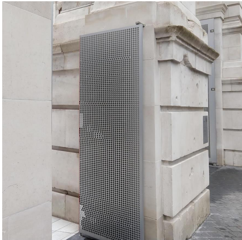
Figure 24, Photo of perforated metal gate attached to Aston Webb Screen.
