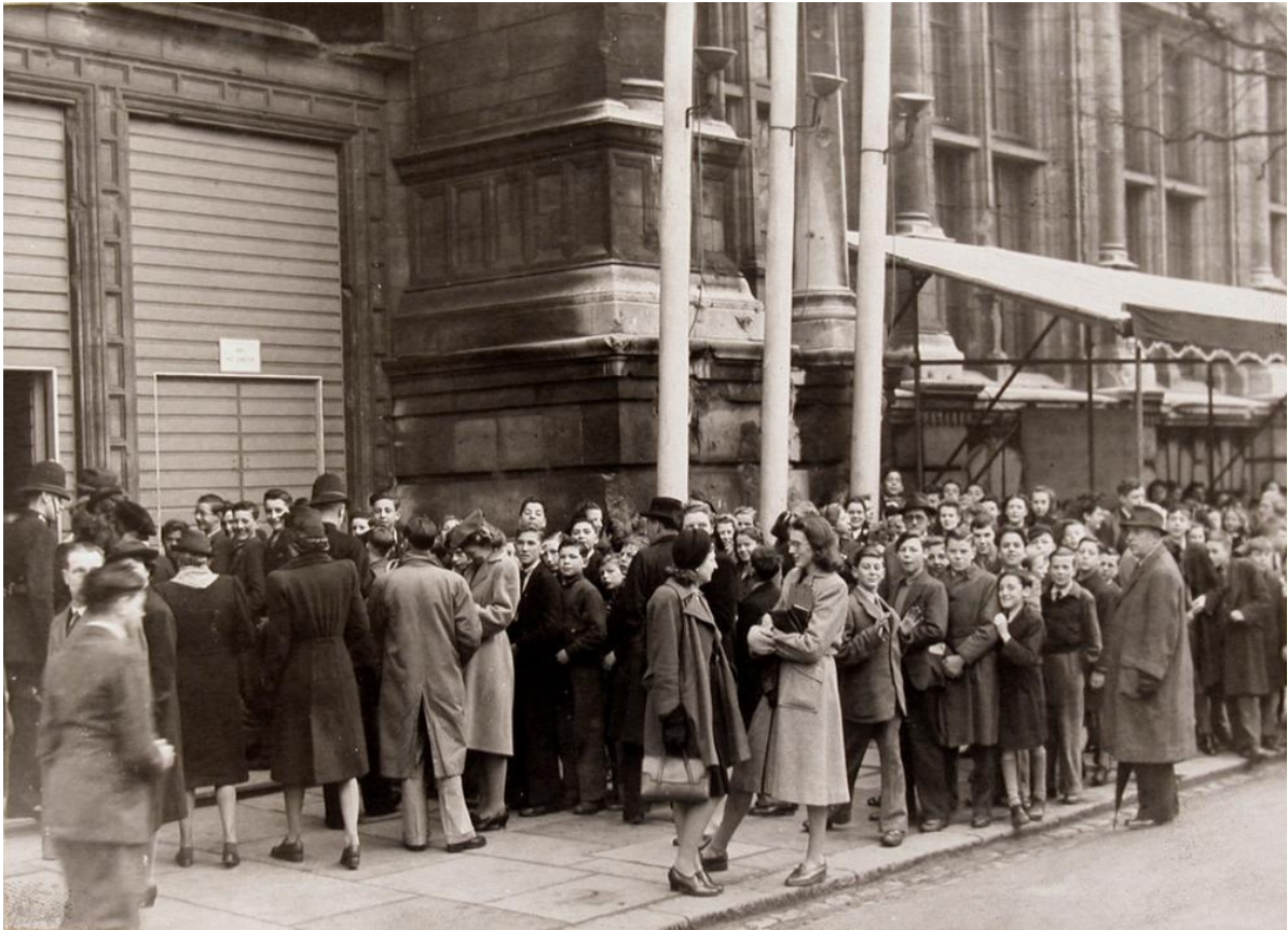
Figure 11, Photo of schoolchildren waiting to enter Britain Can Make It exhibition alongside Exhibition Road façade. Repaired wooden doors, scaffolding, and bomb damage to stonework are all visible in this image.
